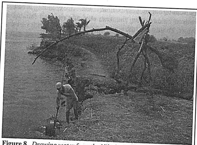
Figure 8. Drawing water from the Nile for irrigation with a shaduf. The shaduf consists of a long beam that rests on a horizontal crossbar in a lever arrangement. On one end of the beam hangs another long beam or a rope to which is attached a bucket. At the other end is a counterweight. The worker pulls down the vertical pole or rope until the bucket goes into the water and fills it. Then the worker pushes it up, and with the help of the counterweight, turns it, and dumps the water into the irrigation canal. Photo credit: ErichLessing/Art Resource.
