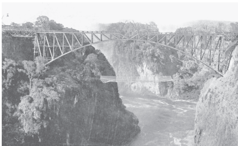
FIG. 4.9. SPANNING THE ZAMBESI RIVER AT VICTORIA FALLS
