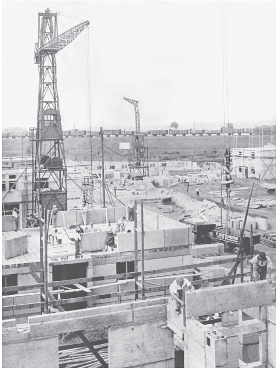
FIG. 6.5. MAY CONSTRUCTION SYSTEM IN FRANKFURT
